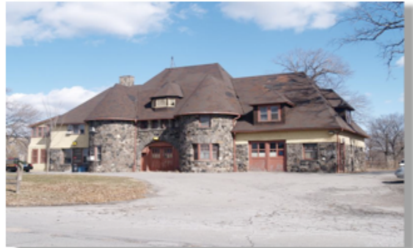
Belle Isle Stables – Now a storage facility
