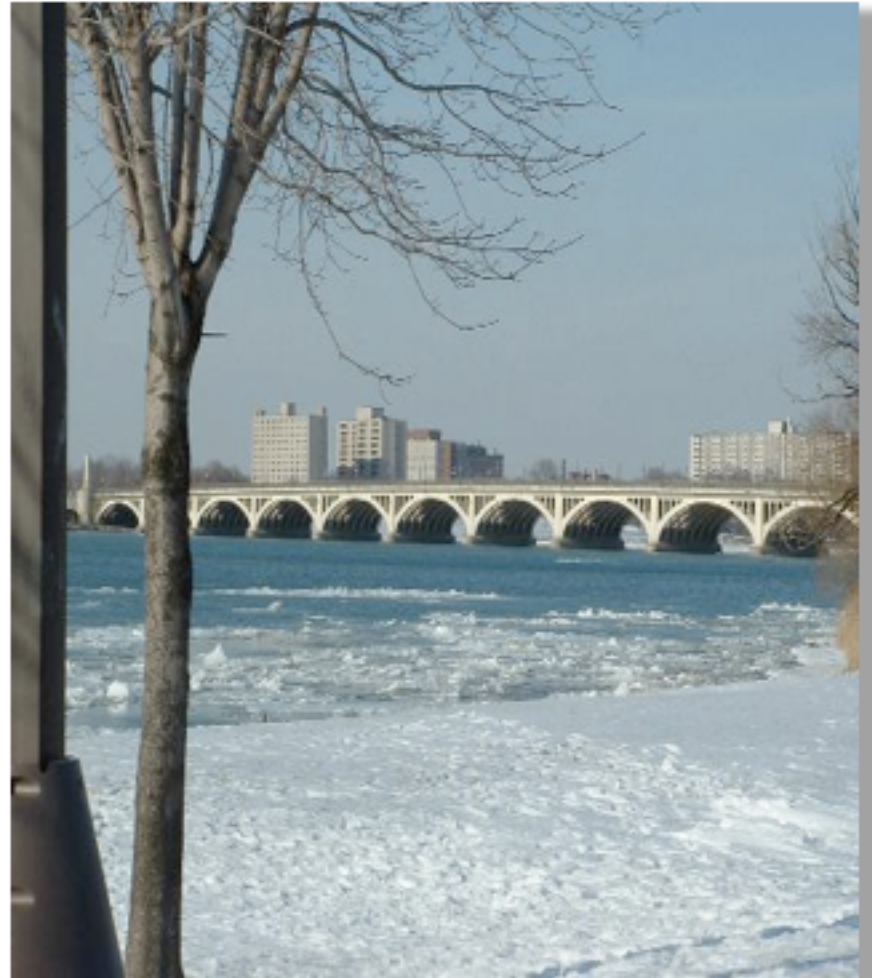
Douglass MacArthur Bridge
