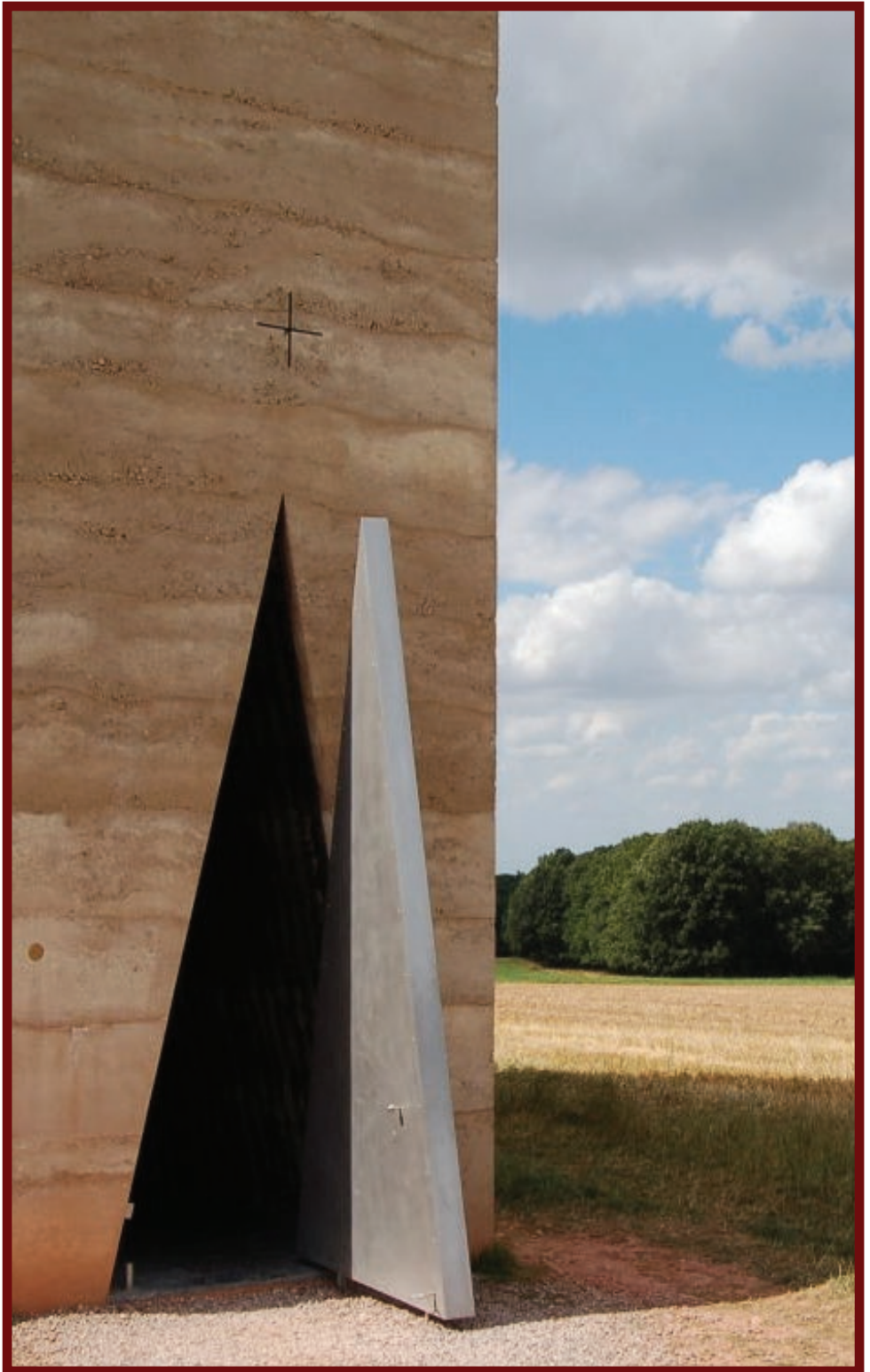
Figure 9.23: Peter Zumthor, Bruder Klaus Field Chapel
