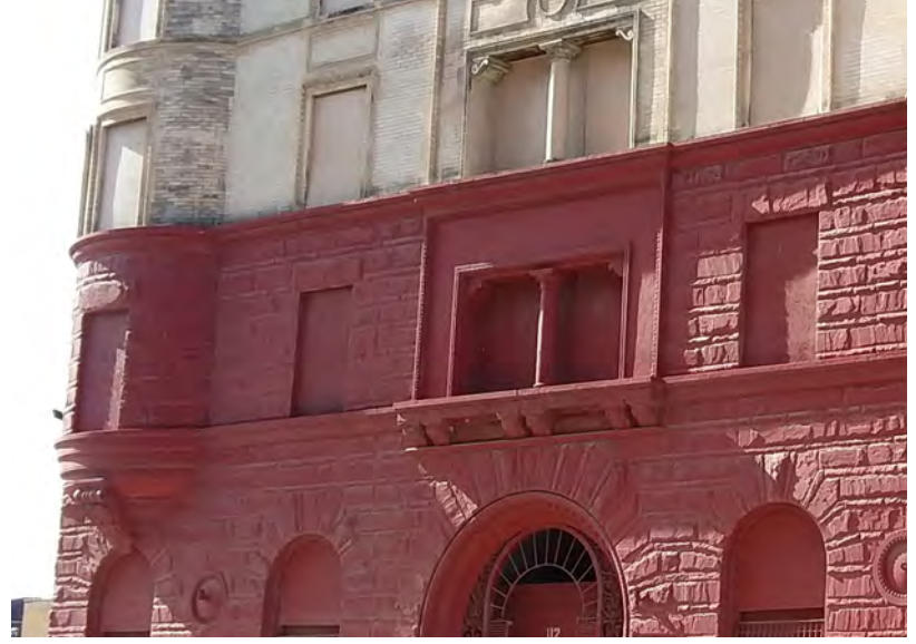
Figure 2.10: Image showing details in windows on the Alhambra Apartments
