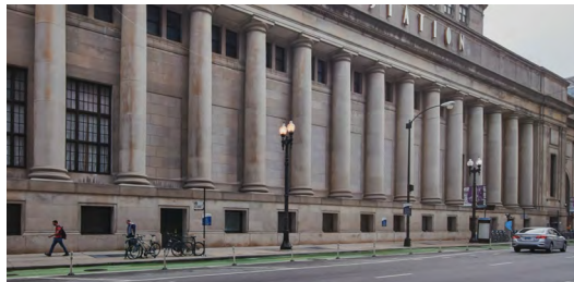
Figure 3.31,3.32: Chicago Union Station on February 2020. Images depict the present state of the Fred Harvey Lunchroom. (22)
