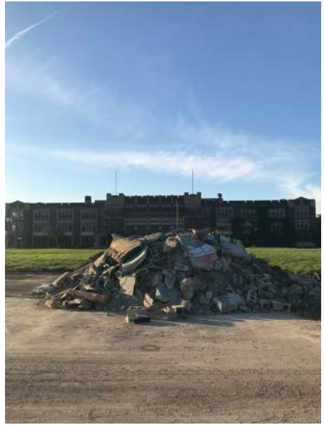
Figure 1.4 ~ The Remnants of The Wig's Demolition
