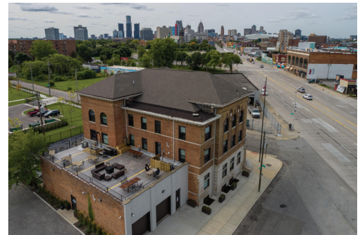
Figure 3.24: Hunt Street Station
