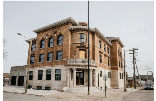
Figure 3.23: Hunt Street Station
