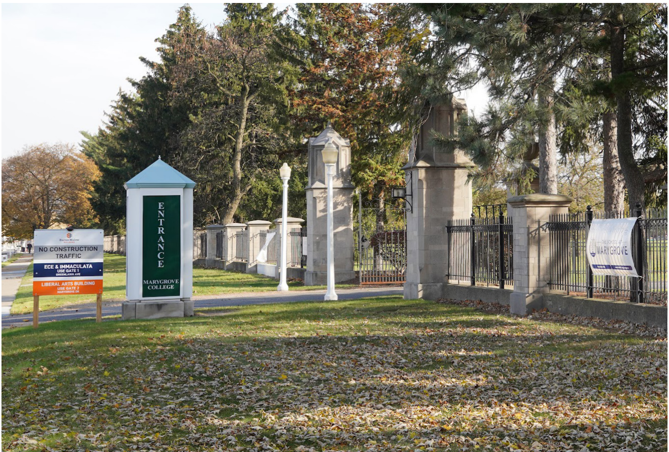
Marygrove Campus entrance with construction signage, Fall 2021
