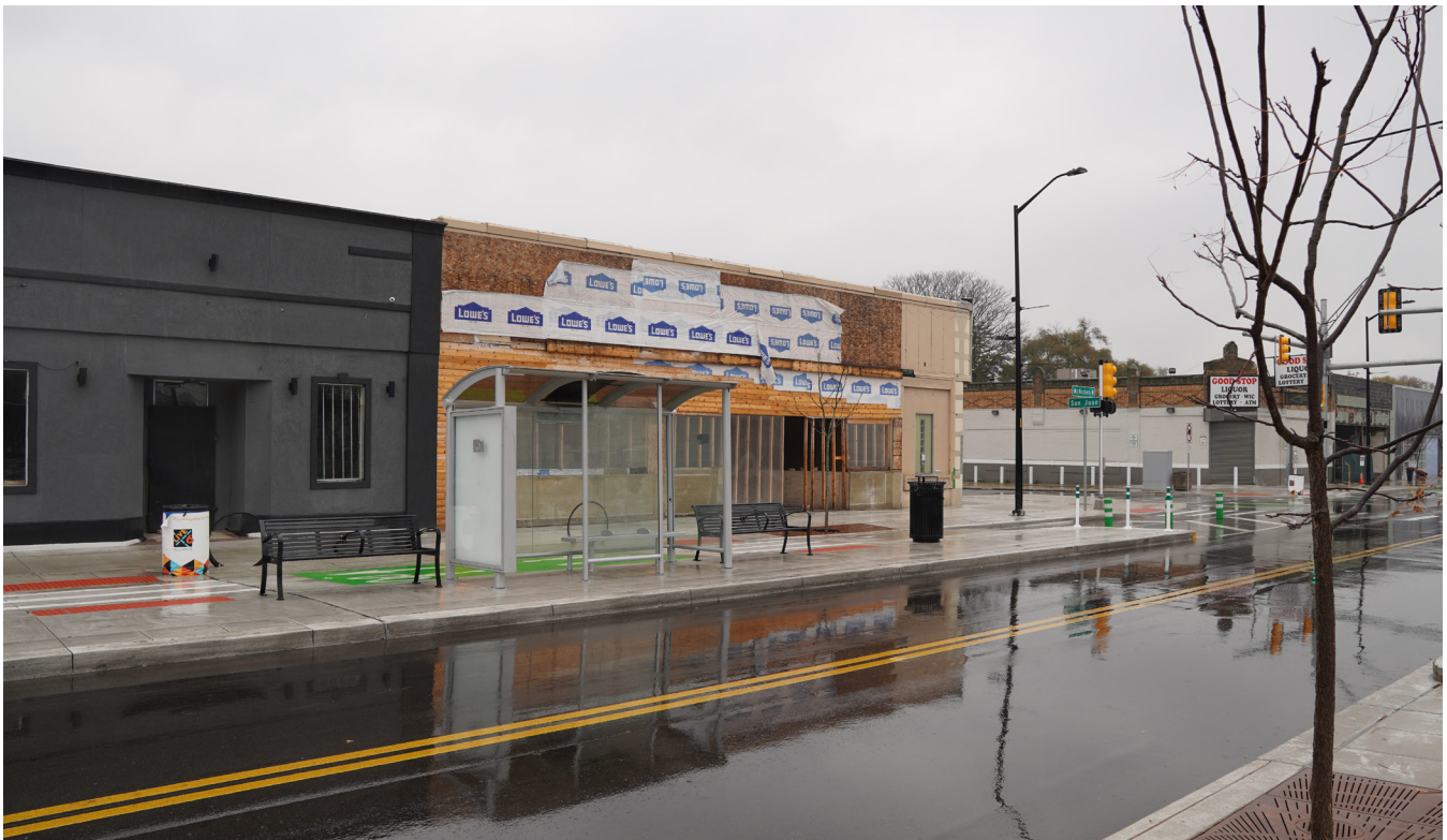
Storefront redevelopment in the Fitzgerald Neighborhood, Fall 2021
