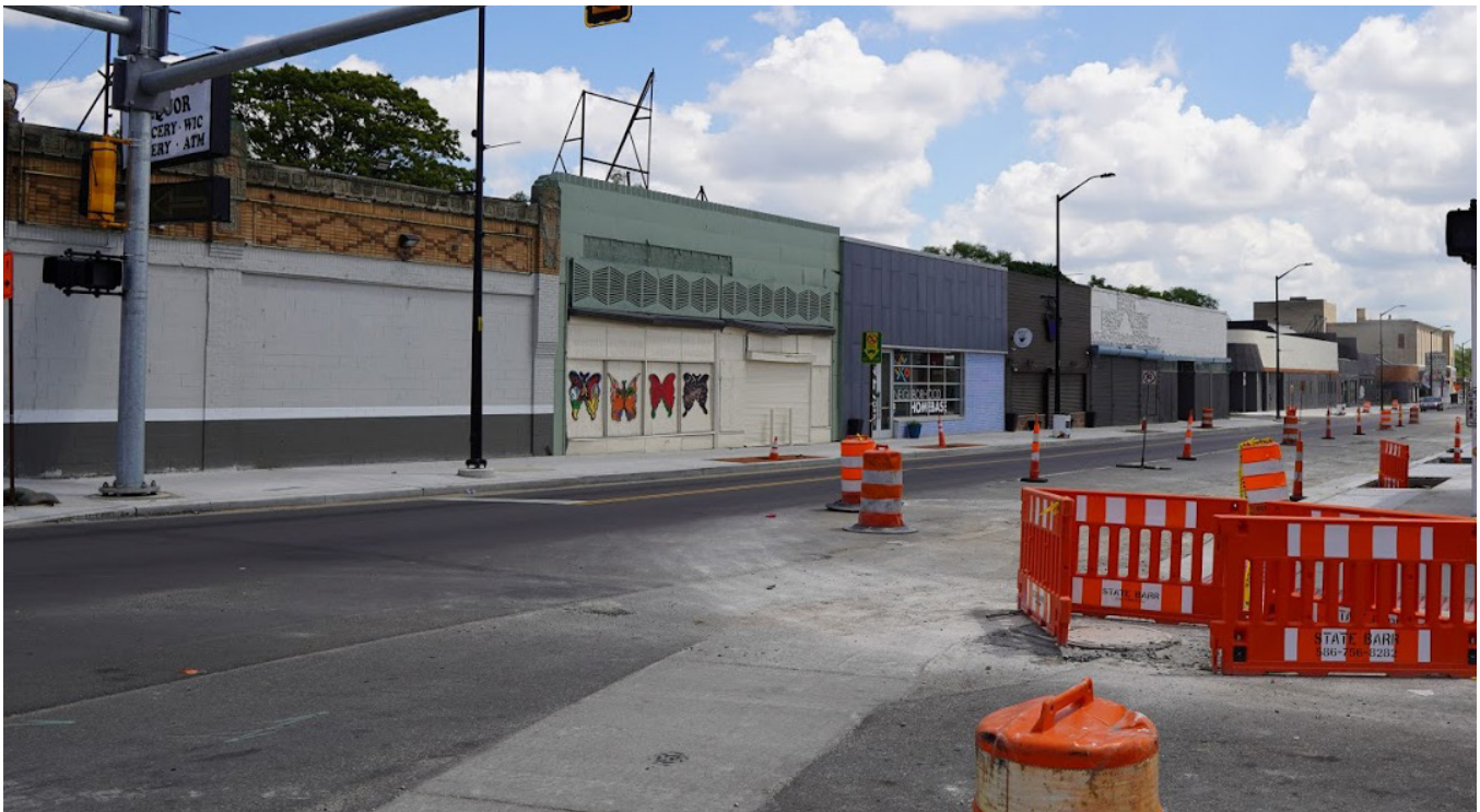
McNichols Streetscape improvements in progress, Summer 2021
