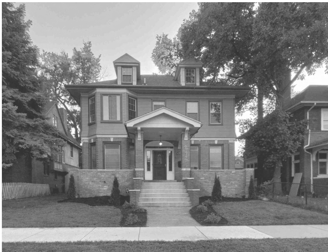
Figure 3.3: DLBA Rehabbed and Ready House
