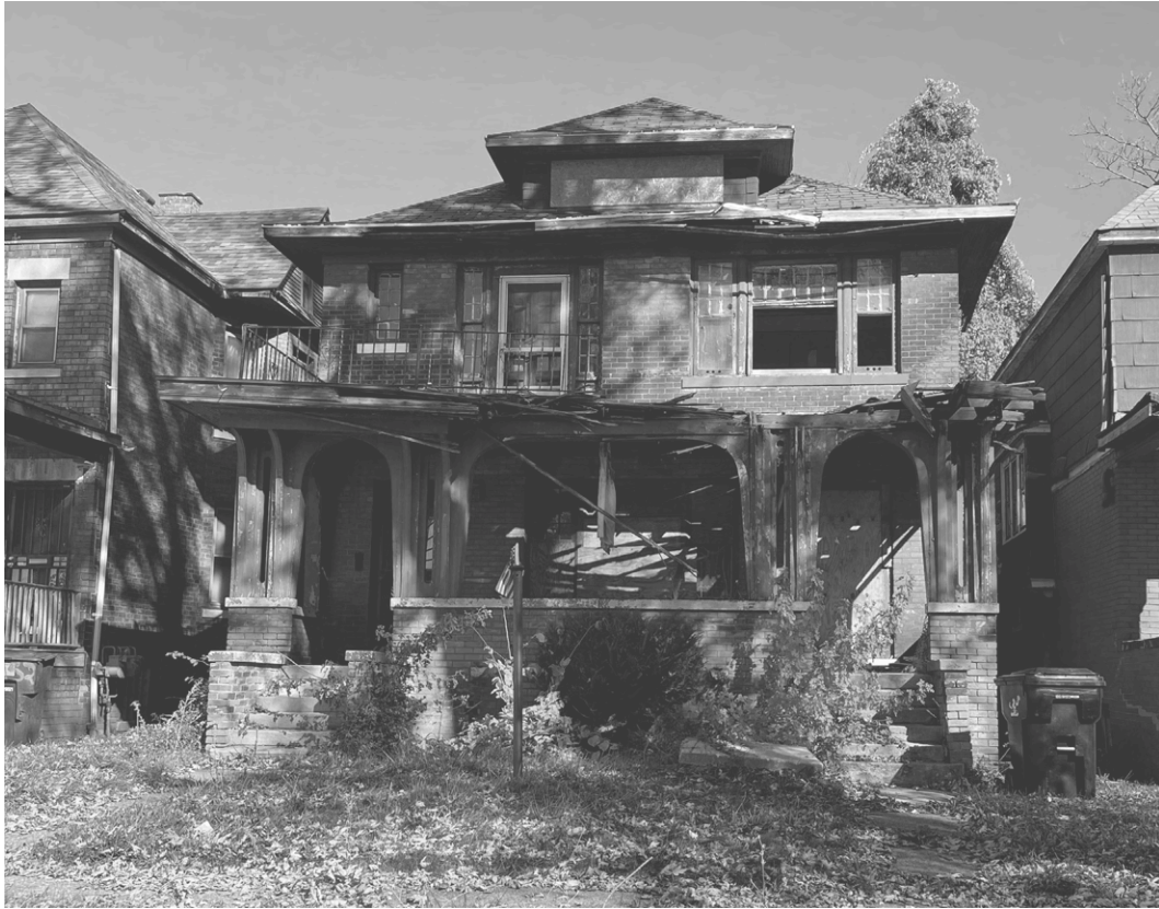
Figure 4.28: Islandview Abandoned house, Duplex
