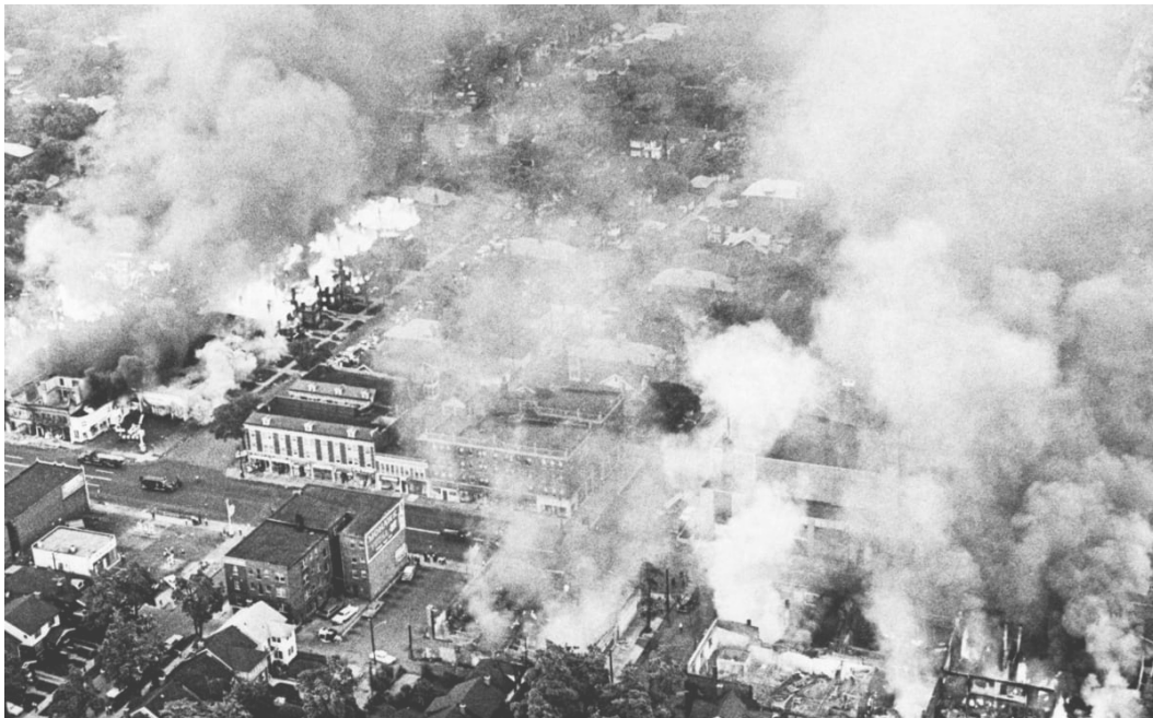
Figure 1.4: Aerial image of riots in Detroit, 1967
