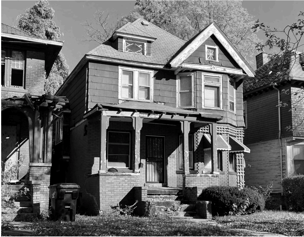
Figure 4.30: Islandview Occupied House, Single Family
