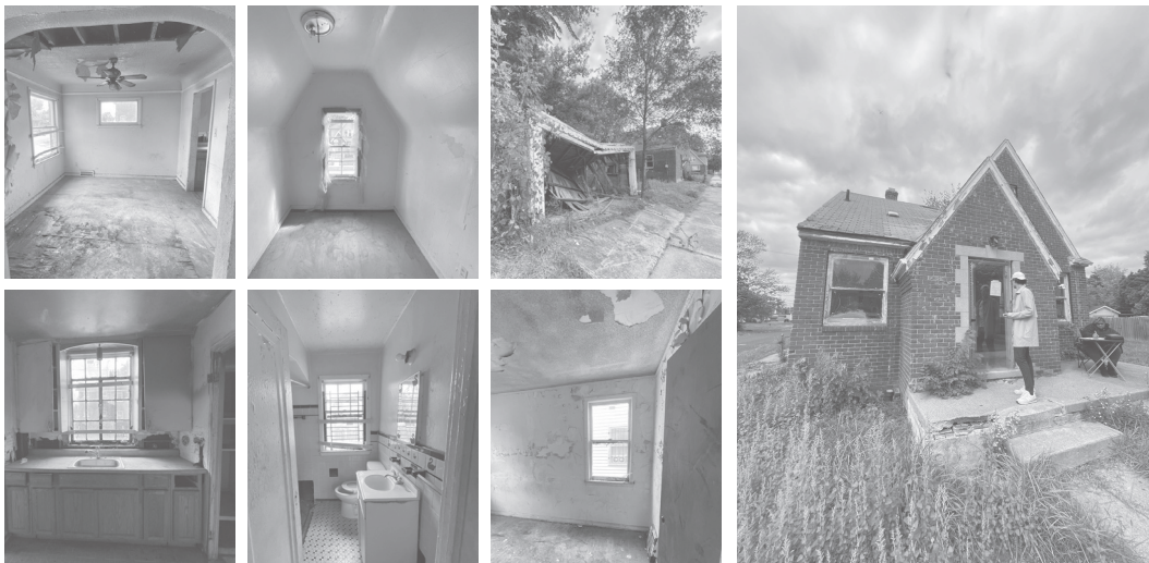
Figures 4.8-4.14: Site photos of DLBA Auction house, located at 12203 Wilfred, Detroit, MI 48213
