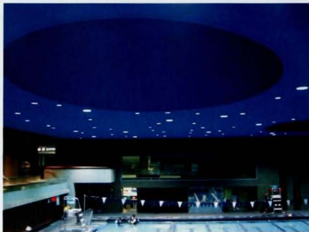
One of the oculi in the roof that allows for natural lighting and ventilation
