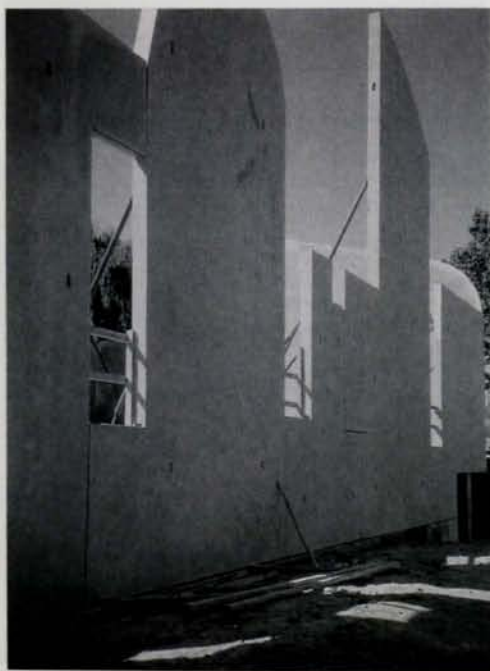
Concrete panels being tilt-up and braced during construction and the final product above.
