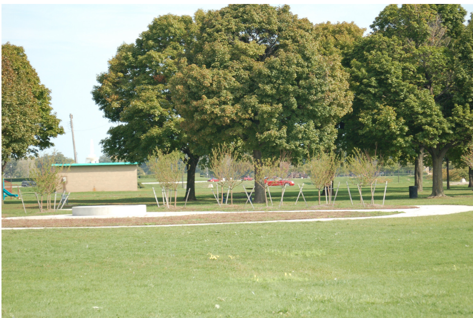
Photograph of the existing restroom on the Apex.
