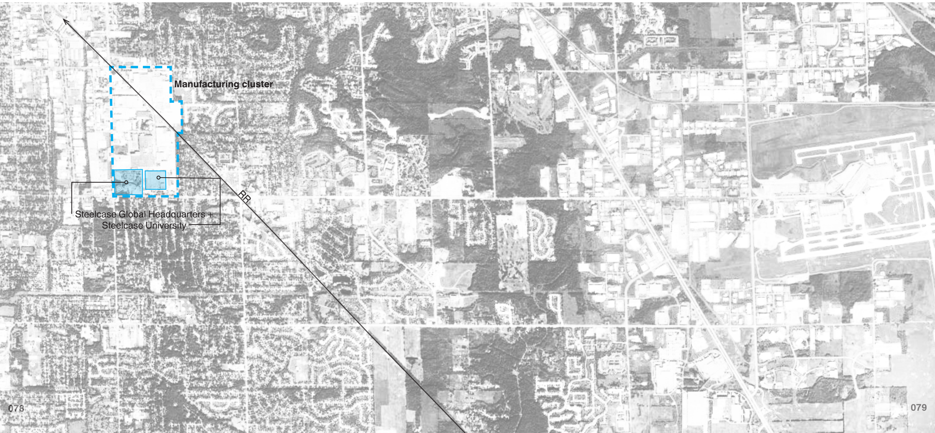
Below Aerial image of Steelcase's global headquarters. Corporate facilities are shaded blue, while the entire manufacturing campus is outlined. The location in suburban Kentwood is accessible to major local infrastructure and is five miles from the city center.
