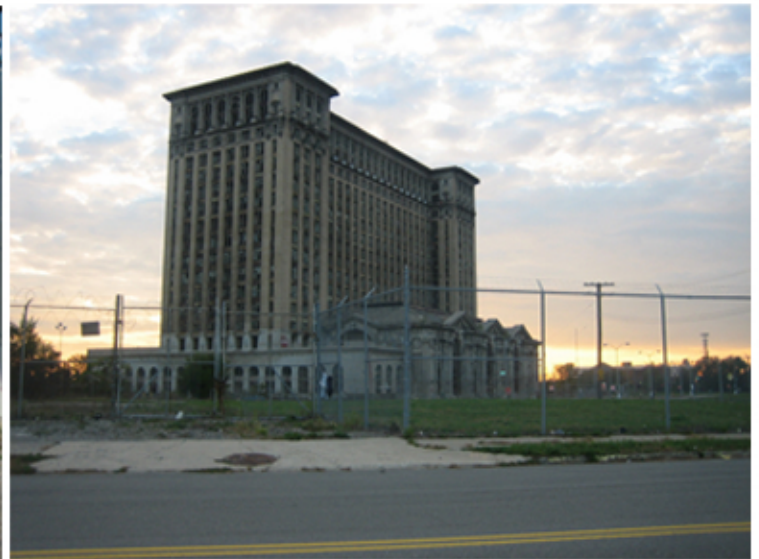
The old Michigan Central Station in downtown Detroit. This once lively structure is now almost in ruins because of abandonment in 1988.
