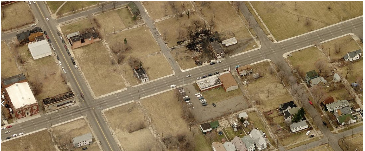
Bird's eye view centered on Forest Avenue shows majority of buildings demolished.
