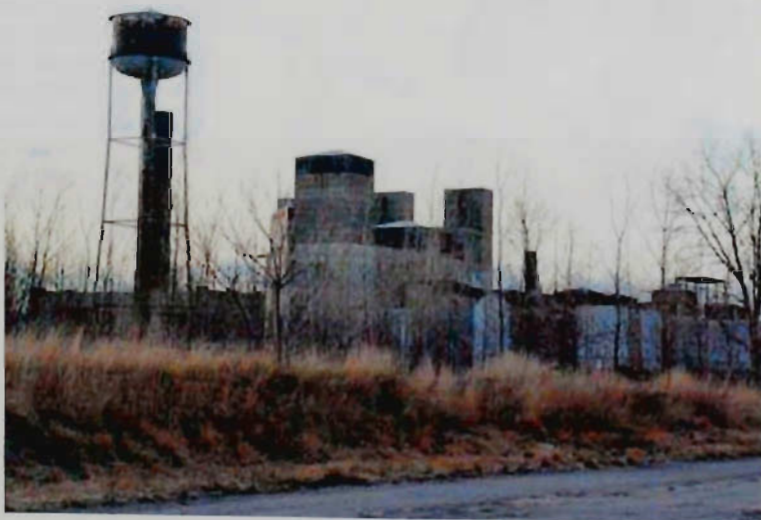
These are some images of the abandoned building on the site. The towers dominate the viewers eye.
