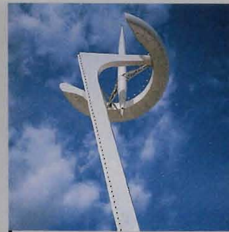
Communications Tower Barcelona, Spain Santiago Calatrava
