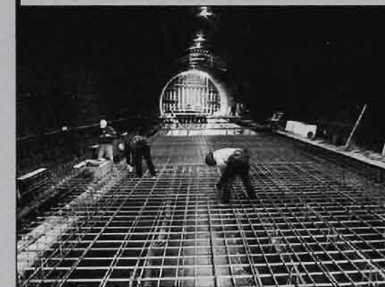
Constructing the "big dig"
