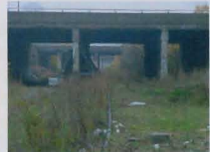
Abandoned Rail Line & Overpassing Bridges
