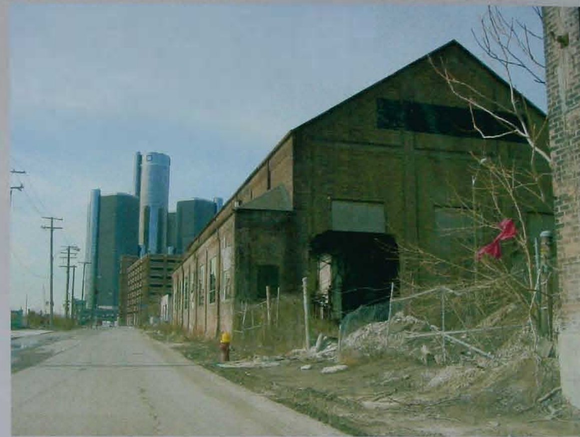
Atwater Street - Crumbling historic structures and streets
