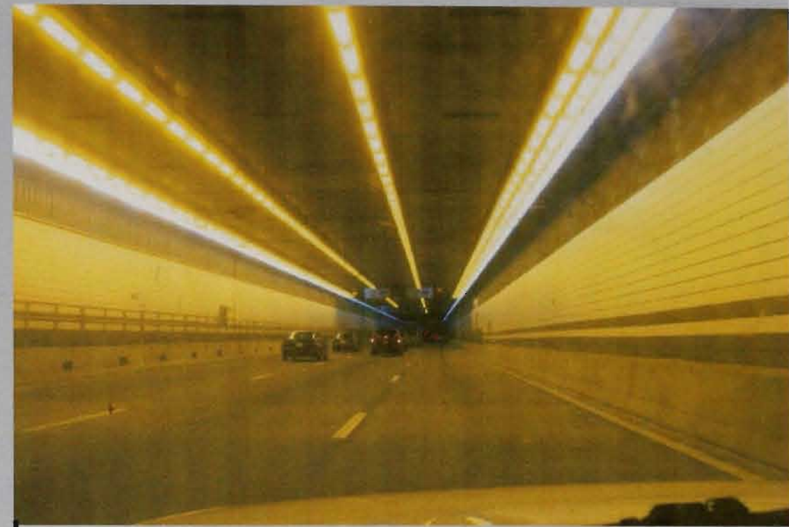
Boston "big dig" Driving underground without a sense of the city
