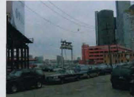
General Motors Parking Lots and Structures
