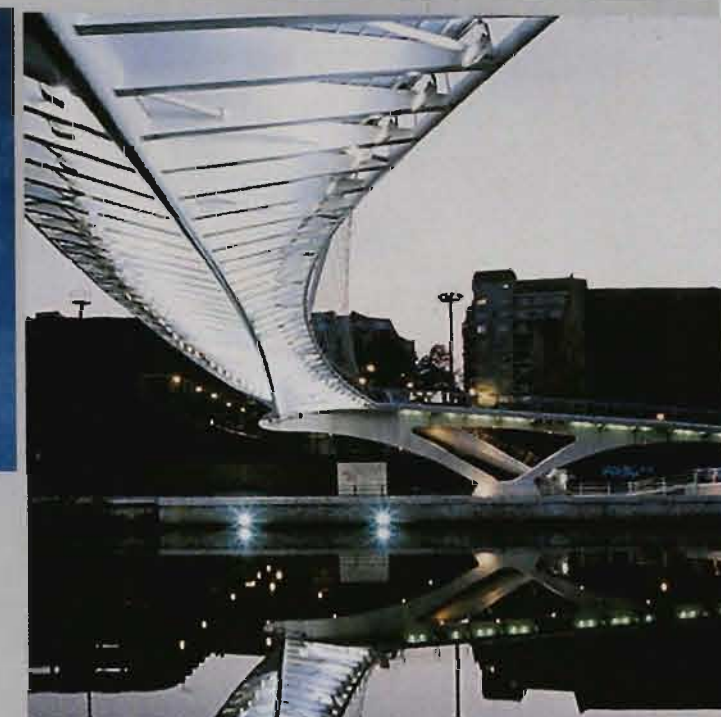
Campo Volantin Footbridge Bilbao, Spain Santiago Calatrava
