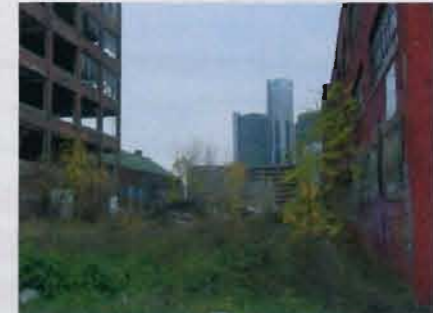
Abandoned Industrial Structures & Rail Line
