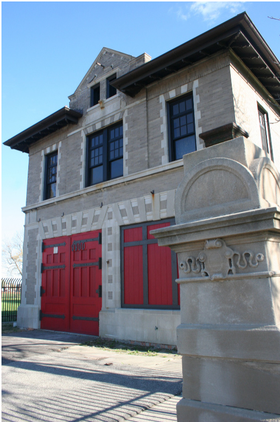
42.2 A former Fire House now acts as support space for neighboring Pewabic Pottery.
