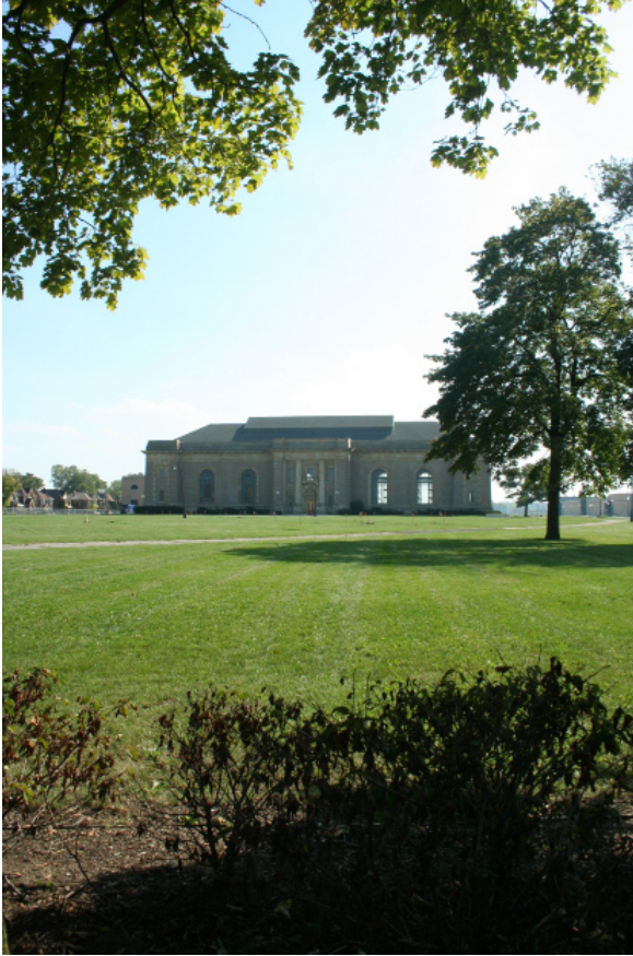
38.1: The Pump House at Water Works Park is an original building.
