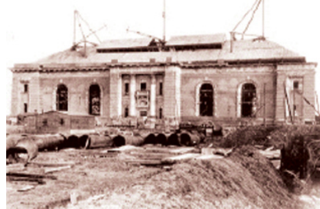
45.1: The Pump house construction being finished.
