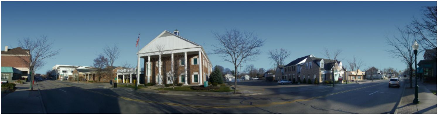
View of Block S from across the South end of Main Street
