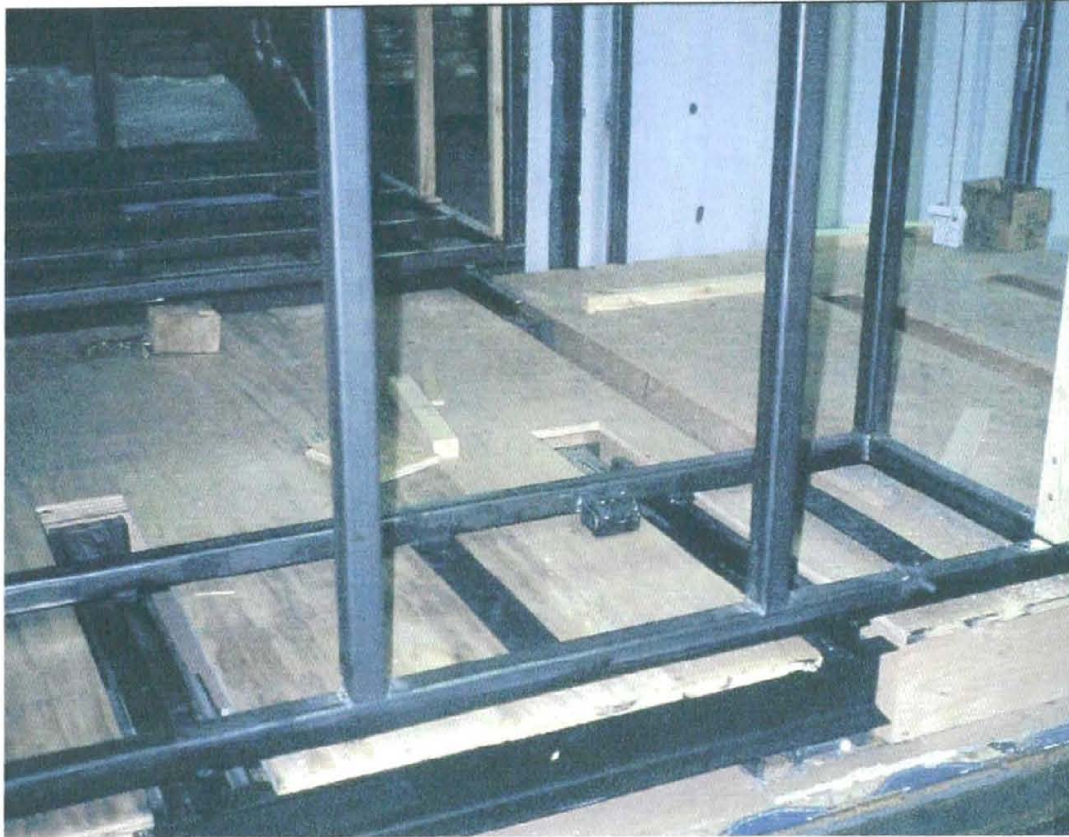
A new floor is built to conceal the working components,
