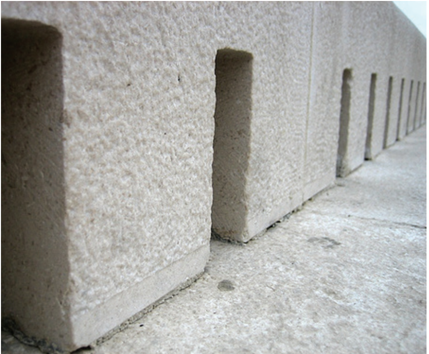
Detail view of the vents cut into the risers of the steps to allow the organ pipes to breathe.
