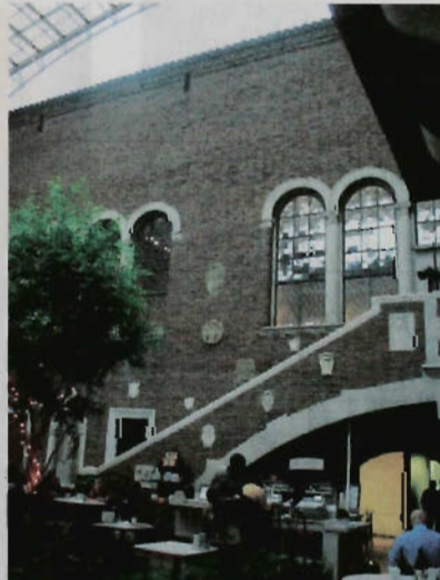
stair to gallery
