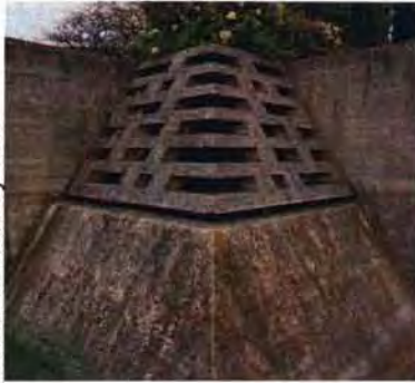
Corner of Boundary Wall
