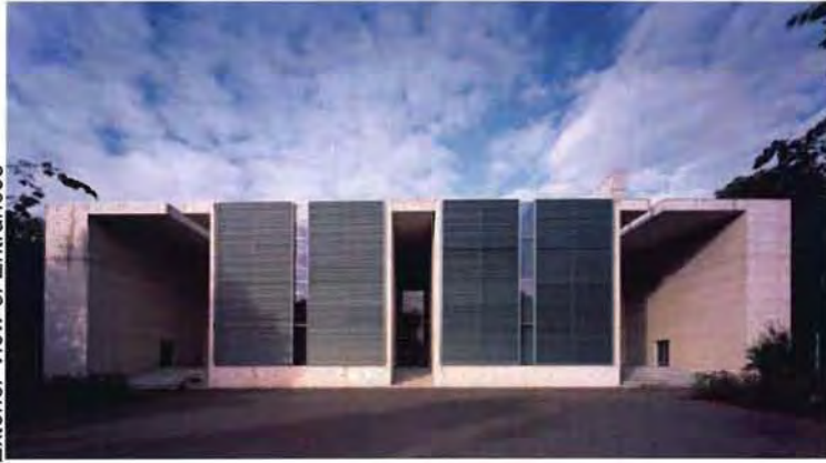
Exterior View of Entrances
