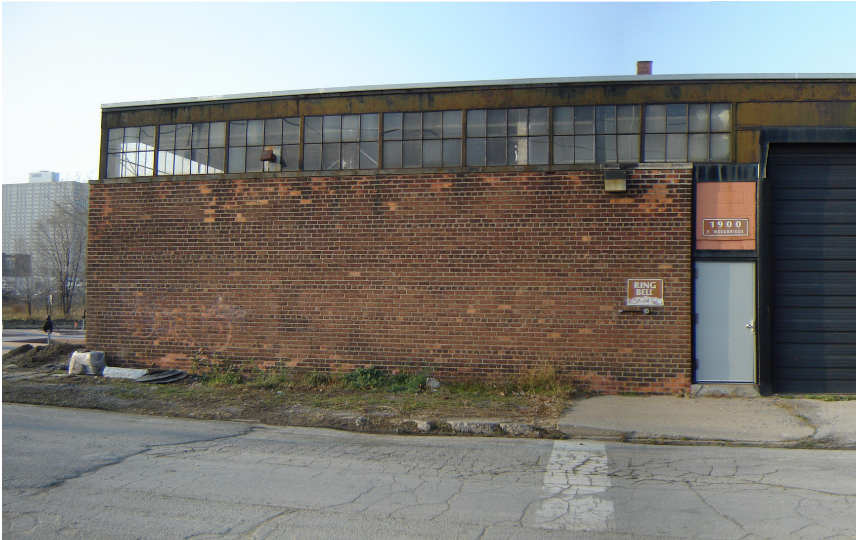
Existing facade along Franklin St. where Museum entrance is proposed
