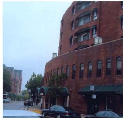
LEFT There is not an issue here of wasted space mediating the street and building frontage. The vertical expression of these buildings at the edge, and their flexibility to follow the street increases the sense of importance. In some cases as shown, the tallest areas are set back to give the street edge a fitting proportion.
