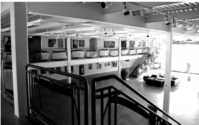
Railing Made From Windshields
