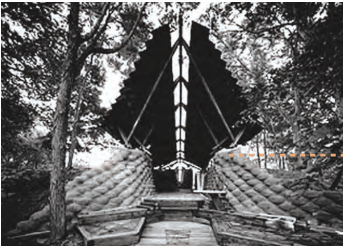
Tires Coated in Stucco
