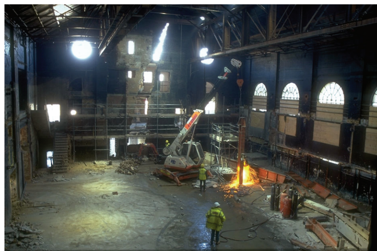
CONSTRUCTION OF THE ALMEIDA THEATER AT GAINSBOROUGH HAWORTH TOMPKINS
