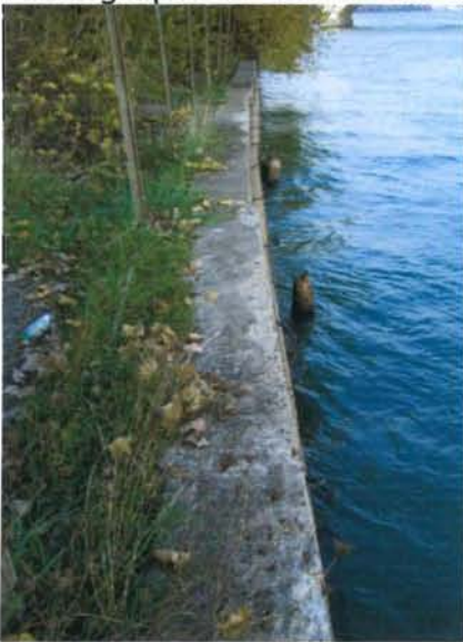
Photographs of site in current condition
