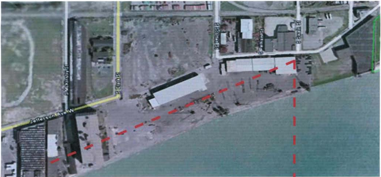
Site B Location-Clark St., Detroit, Michigan
