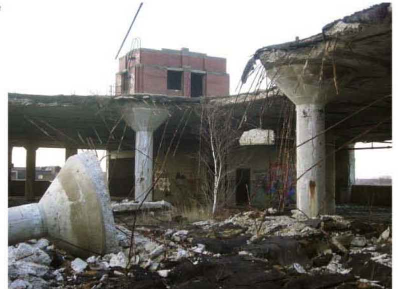
Collapsed roof of warehouse
