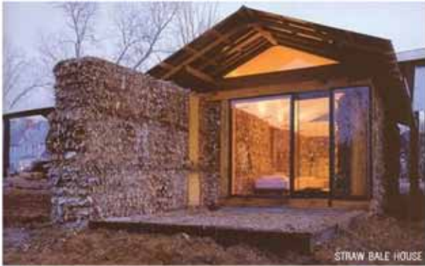
STRAW BALE HOUSE
