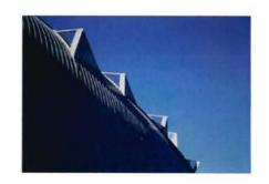
AN INTRICATELY DETAILED SKYLIGHT SYSTEM UTILIZING THE FORM OF THE BUILDING ALLOWS FOR BRIGHT, NATURALLY LIT SPACES THAT WILL NOT DAMAGE THE WORKS OF ART ON DISPLAY. THE SUN'S HARSH ULTRA VIOLET RAYS ARE REFLECTED OFF THE SKIN OF THE BUILDING AND NOT PERMITTED TO TRANSMIT ANY HARMFUL LIGHT INTO THE PHOTOSENSITIVE GALLERIES.
