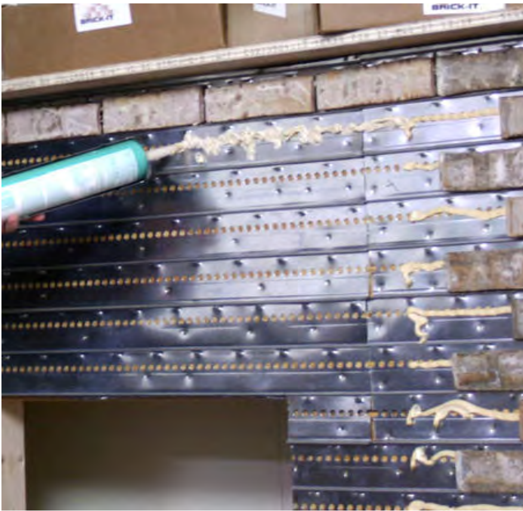
There are various installation methods for brick tiles. These particular installation method includes a metal track for the tiles to rest on.
