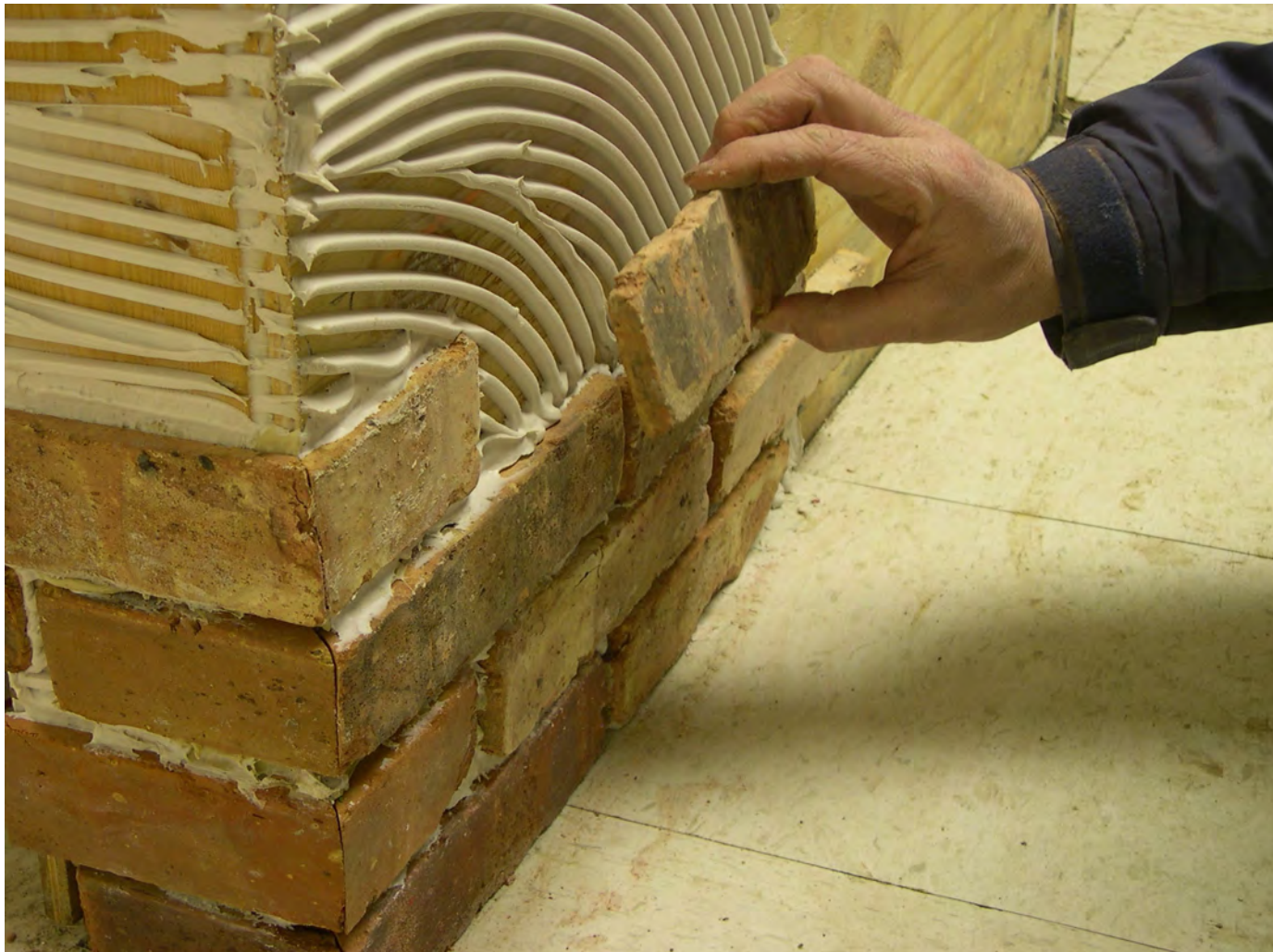
Brick veneers are clay tiles, usually \frac{1}{4} " or \frac{1}{2} " thick, applied on the exterior of a building. They are typically used to mimic real brick and cost less
