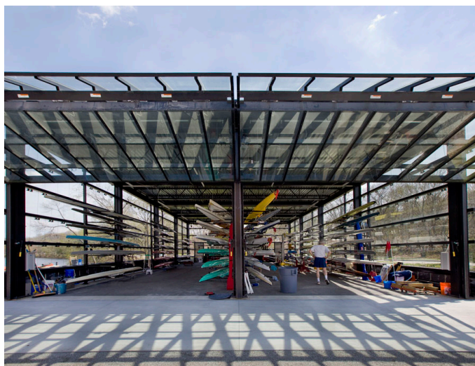
Glass shingle boat storage
