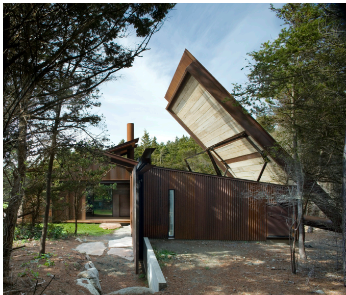
bathhouse roof open
