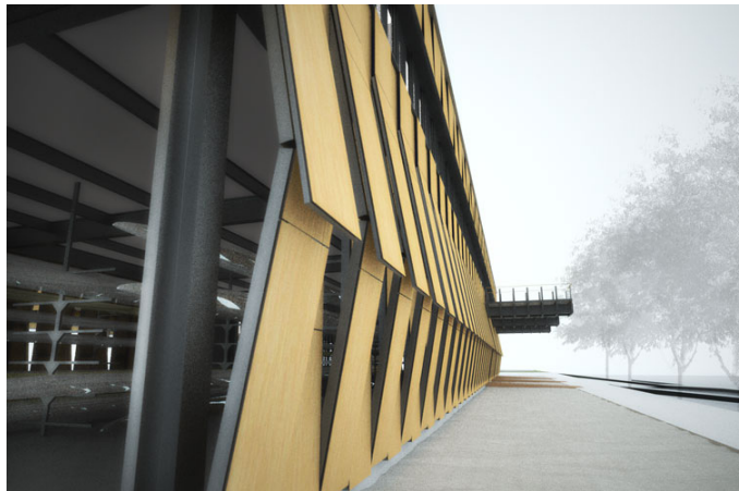
Louver panels open
