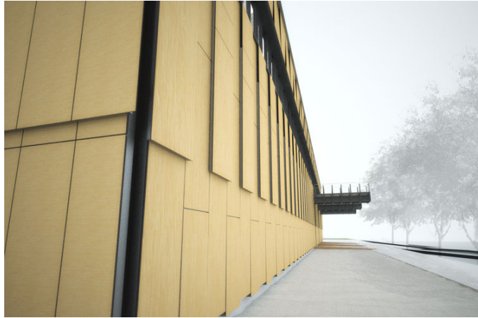
Louver panels closed
