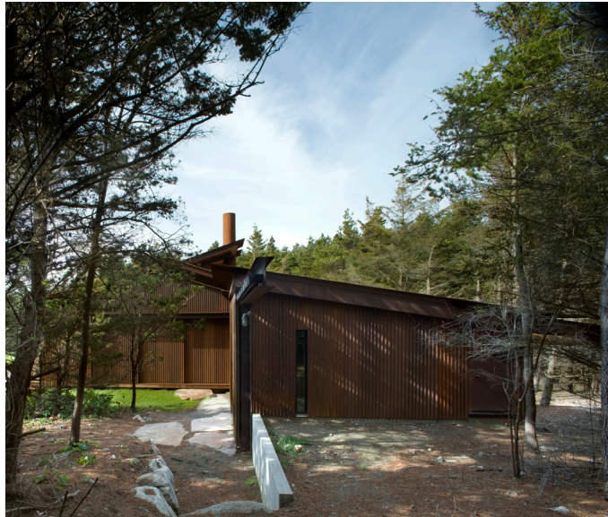
bathhouse roof closed
